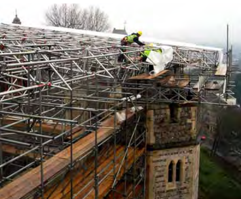
Scaffolding being erected over Canons' Cloister
