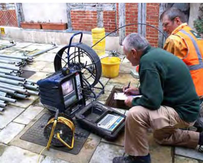
Detailed inspection of underground services in Canons' Cloister
