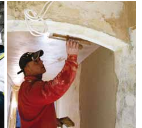
Plastering the ceiling in the basement corridor
