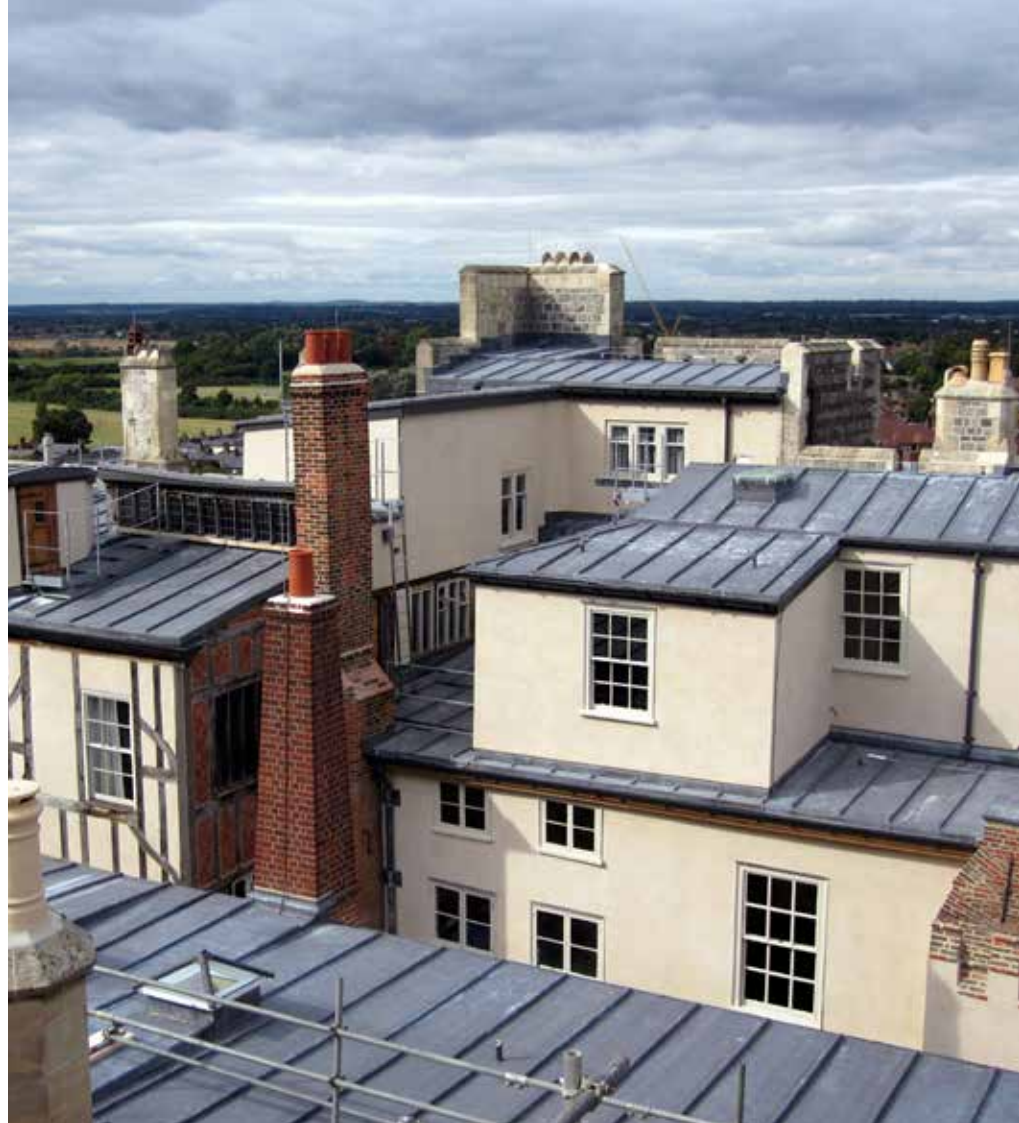
New lead roof as part of the full refurbishment
