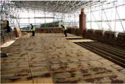
Paul Webb Roofing removing roof boarding over the Dean's Study.
