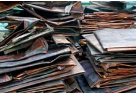
Old copper roofing being removed for replacement in lead.
