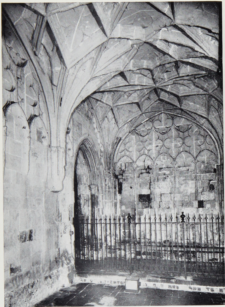
Plate IV. The Porch below the Aerary built in 1353-54. Note the four-centred section of the vault.
