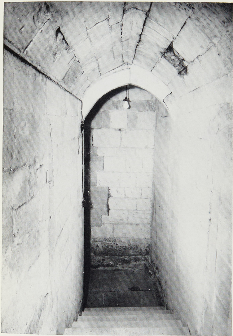
Plate I. The Tresaunt, with its chamfered cross-arch and pointed barrel vault; original masonry of 1240-43.
