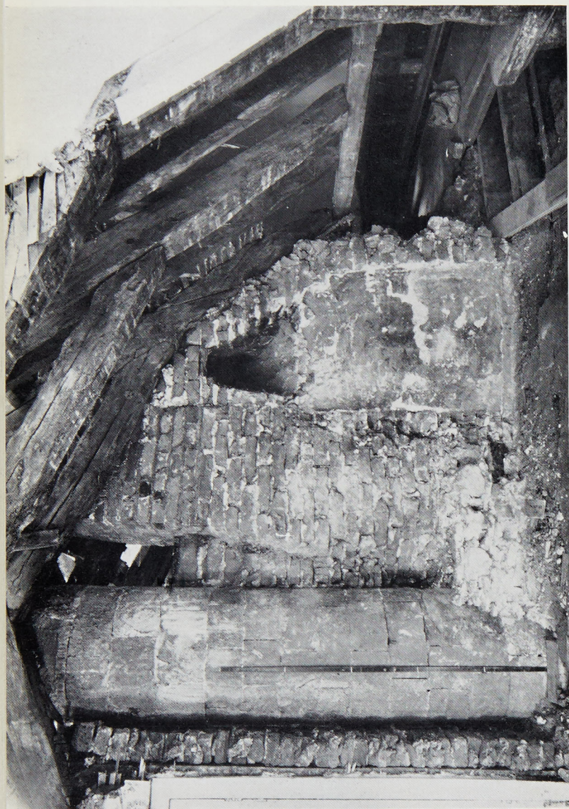
PLATE IV Circular Chimney on the second floor of No. 25 The Cloisters, within scissor-beam roof. On the extreme right an unaltered roof truss can be seen with the ashlar piece rising from the cornice. (Photograph taken in 1965 before restoration.)
