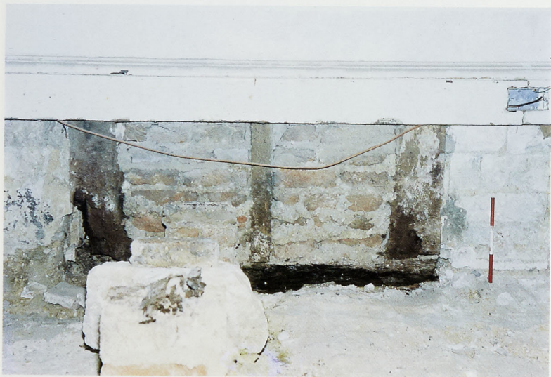
Plate 15. Timber and brick infill to niche in south wall.
