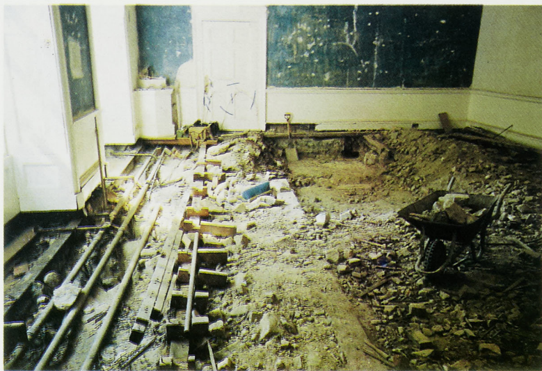
Plate 3. RG2 Sitting Room. Loose building rubble revealed below suspended floor.
