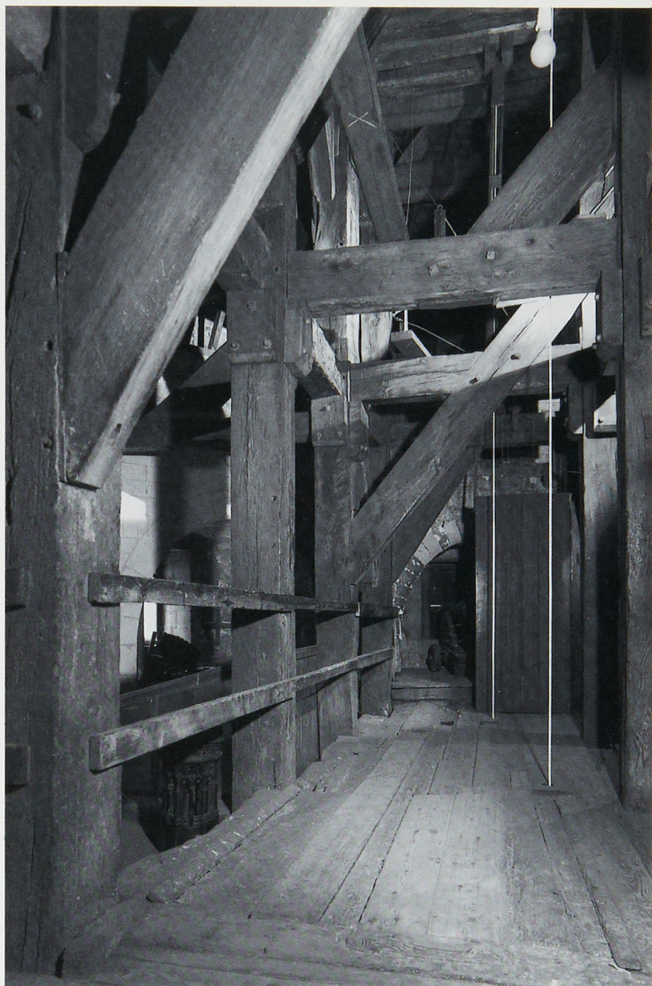
PlateX: The first stage of the Curfew Tower, showing four of the outer (on the left) and two of the inner posts of the massive fifteenth-century frame. Note the bell-ropes running up to the bell-frames above, and the new bolted-in timbers half way up. Thirteenth-century masonry can be seen in the background.
