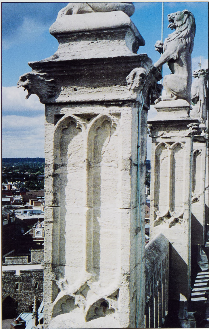
Plate VIII: Pinnacle on the south side of the Chapel, showing serious erosion, especially of the carved heads (see page 198).
