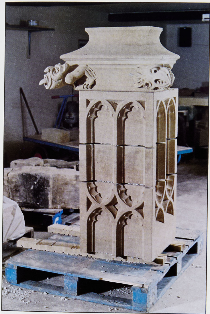
Plate IX: Newly carved stones for the pinnacle are assembled in the workshop.
