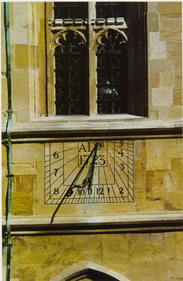
Plate III. The newly-refurbished sundial on the Schorn Tower. Some of the stonework repairs are visible on the window above.
