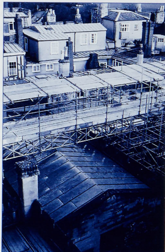
The scaffolding gantry flying over the Chapter Room.
