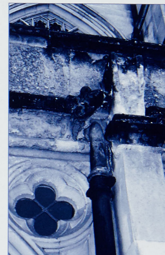
Inadequate rainwater outlets via carved stone gargoyles.
