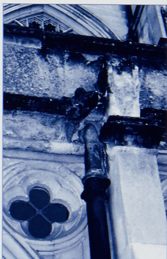
Inadequate rainwater outlets via carved stone gargoyles.
