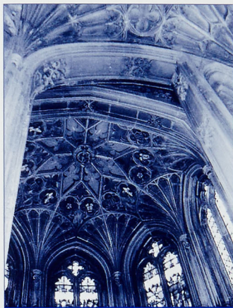
figure 1: The rooflines of the Urswick Chapel (north-west chapel) and the Nave, showing evidence of the curtailing of the original design.
