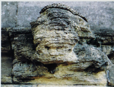
A corbel sculpture weathered to the point where no significant marks of the original carving remain.
