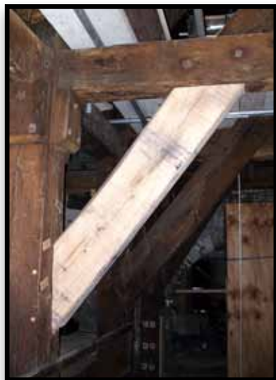
Figure 3: Newly-inserted timber brace.
