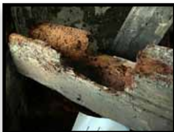
Figure 1: Evidence of death-watch beetle attack.
