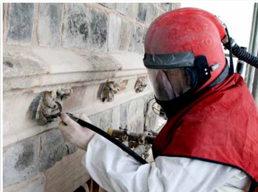
Figure 9: Detailed cleaning of upper string course of curtain wall, March 2009.
