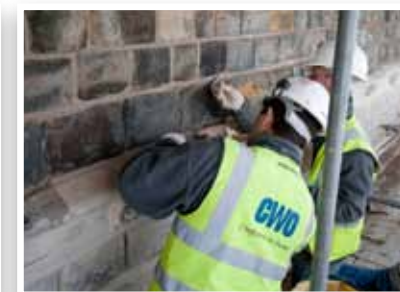
Figure 8: Stone pointing on the curtain wall, January 2009.
