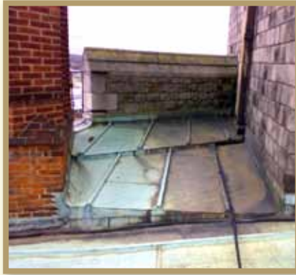
Figure 3: Copper roof on the Canons' Cloister in great need of repair.
