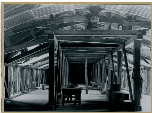
Figure 2: Quire Vaulting under repair.
