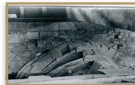
Figure 4: Quire vaulting being reset, and end of repaired tie-beam.
