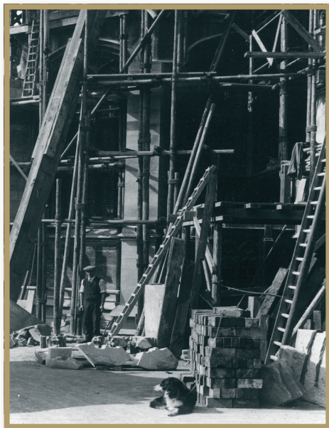
Figure 5: South Transept, shoring and scaffolding for new buttresses
