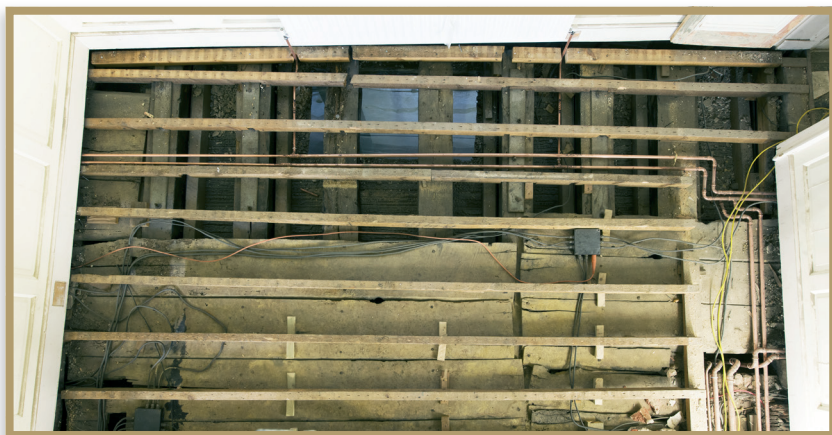
Figure 4: The drawing-room floor of No. 5 (south at top). Under 1960s softwood joists, the mediaeval floor boards are clearly seen, supported on the original joists. The remains of the hearth are just visible bottom right.
