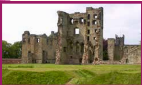
Figure 3: The massive tower of Ashby-de-la-Zouche.
