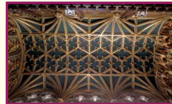
Figure 5: The vault over the Hastings chantry.
