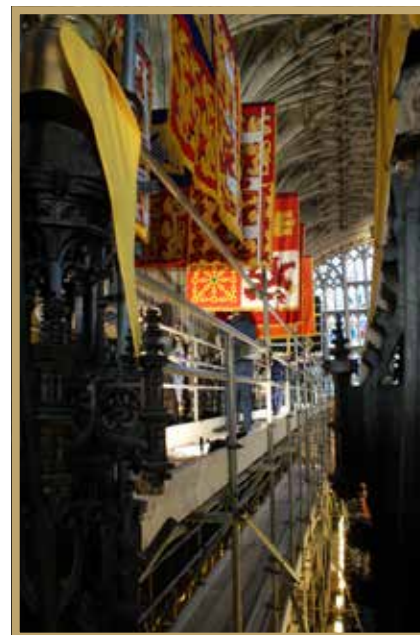
Figure 5: The scaffolding for the 2017 high-clean in the Quire.
