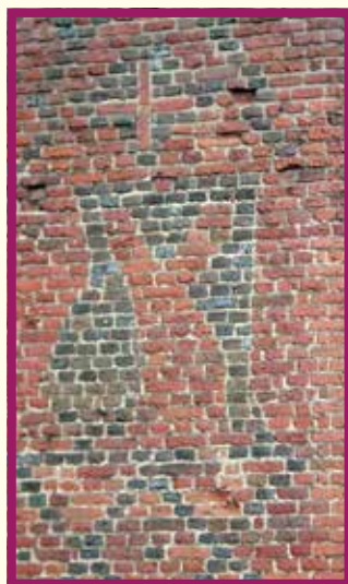
Figure 2: The Hastings Maunche (sleeve) in black brick on the gatehouse at Kirby Muxloe.
