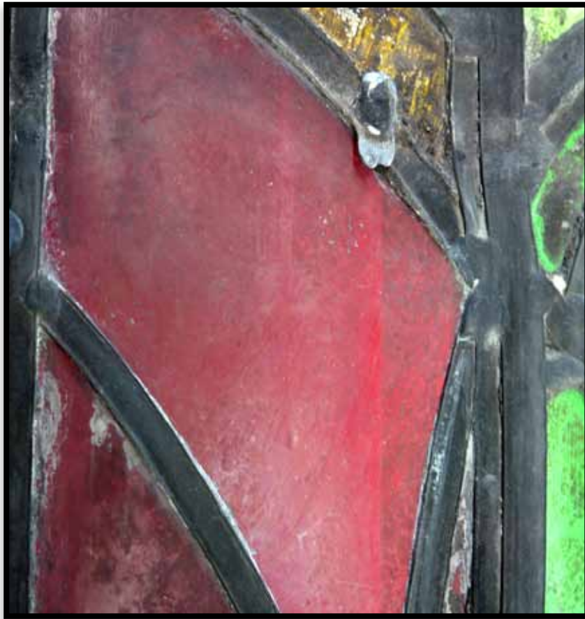
Figure 4: Detail of panel showing considerable scaling.
