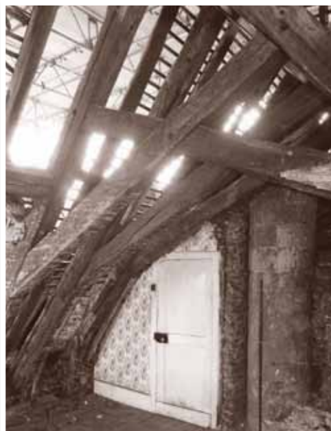
Figure 5: Remaining scissor-braced roof in No. 25, uncovered during work in 1965.
